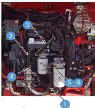
1. EFP inlet pipe 2. Secondary filter inlet pipe 3.
