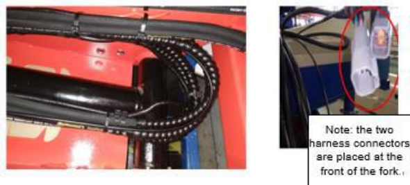
Fig. 4.48 Installation of first layer pipeline
