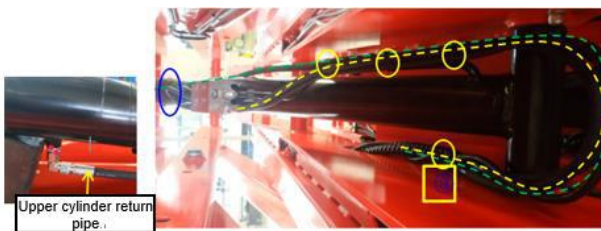
Fig. 4.90 Installation of third layer pipeline
